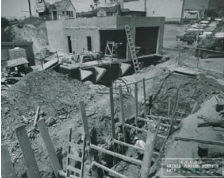
Orinda Pumping Station in 1960
